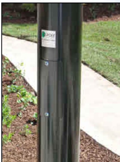
Powder Coated over Hot Dip Galvanising
